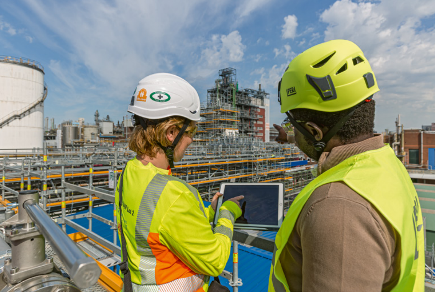
New construction of vitamin A plant, BASF (Germany)
