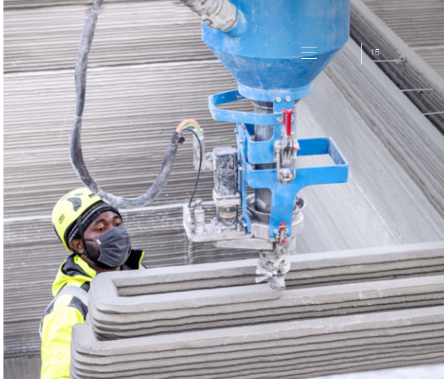
A new, innovative way of building: 3D Construction Printing
