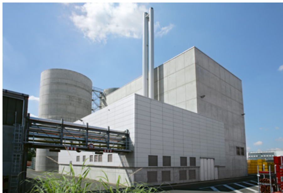
Biomass power plant at the Weissenhorn site
