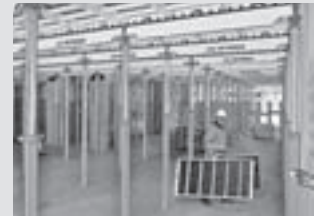
Slab Formwork
