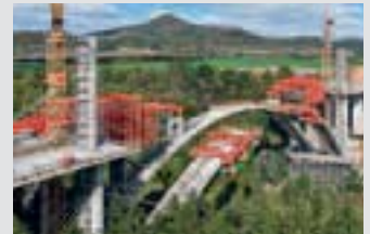
Bridge Formwork
