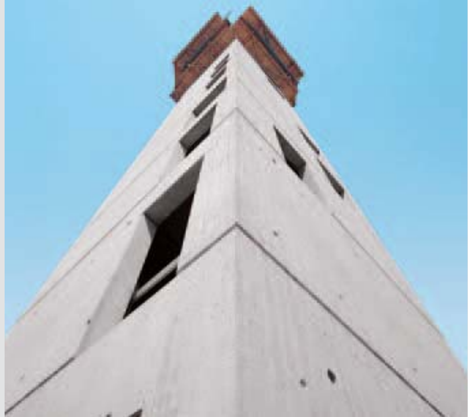
Attractive looking concrete finish with rough vertical board finish.
