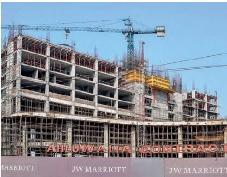
Multi-storey Hotel and Service Apartment with VARIO VT 20 and RCS/VARIO rail climbing formwork systems used for lifting core walls.
