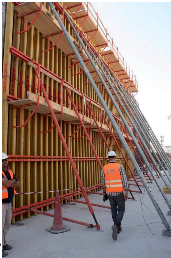
Several working platform levels are required at great heights.
