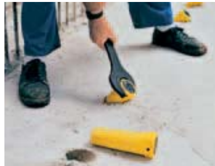
The Leading Anchor Coupler is removed using the Single-Ended Spanner SW 70.
