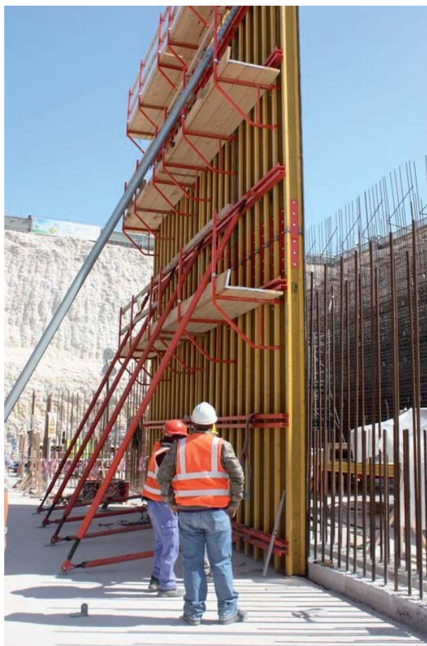
8.00 m high Metro station walls extended with extension splice for VT.
