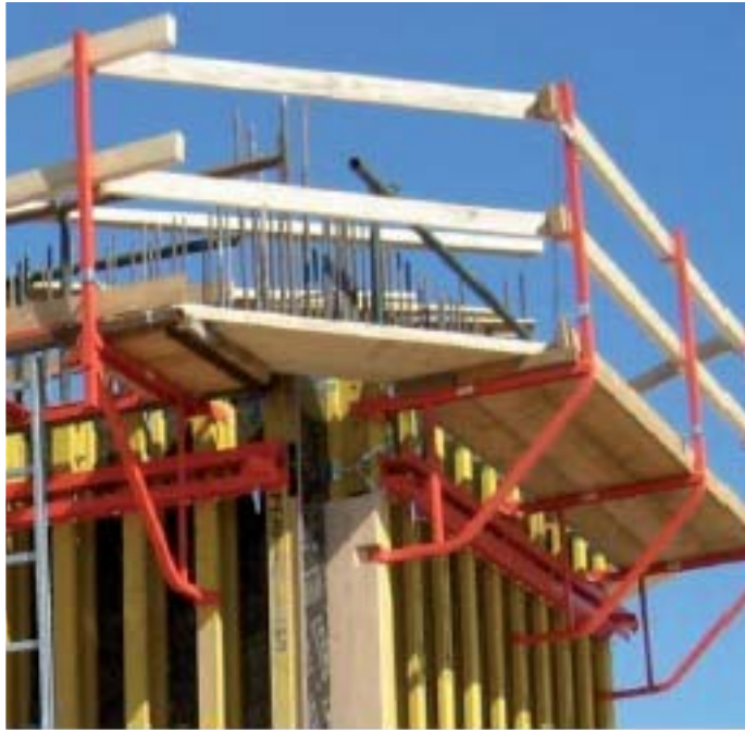
A correctly assembled concreting platform complete.
