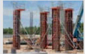
Column Formwork
