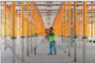
Slab Formwork
